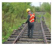
**4.** Pull the rope taut and clamp the paddle to the rail as in step 1.
