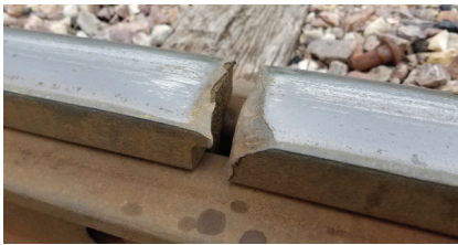
Battered Rail Ends
