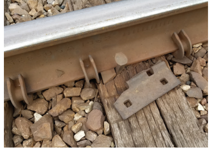
Broken Tie Plate
