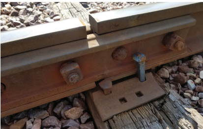
Spikes Loose Near Joint Bars
