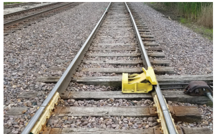
Properly Ballasted Track
