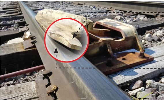
Previously Damaged Derail
