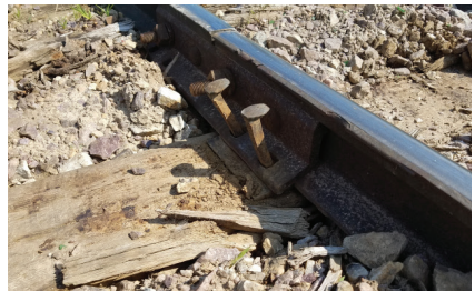
Spikes Loose Near Joint Bars
