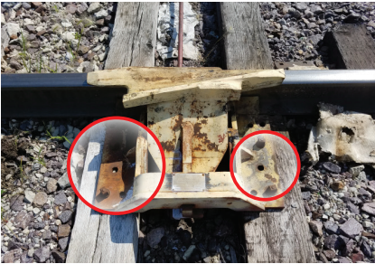
Missing Spikes/Screws
