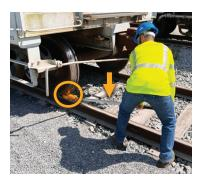
3. Repeat this process until the rail car is in the desired location. Set the rail car brakes and install wheel chocks.
