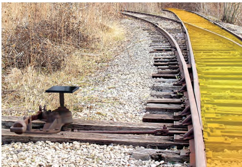
Left-hand switch, viewed from “switch point” end. Mounting platform is in place and ready for sign plates.
