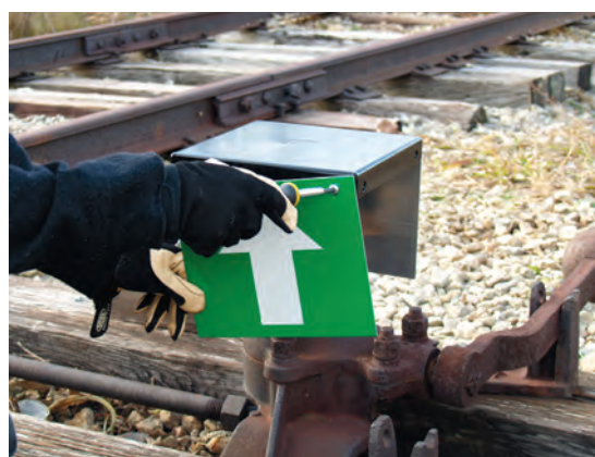
Then install the other green plate on the opposite side of the platform (the “frog” side).
