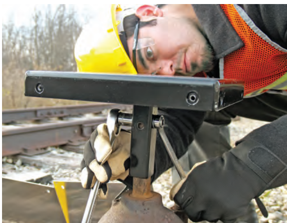
Left-hand switch, viewed from “switch point” end. Mounting platform is in place and ready for sign plates.
