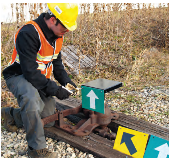
Then install the other green plate on the opposite side of the platform (the “frog” side).
