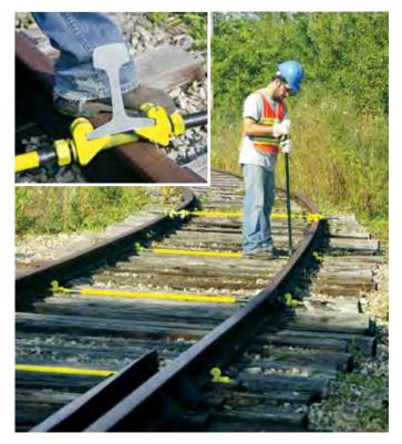
A simple preventive measure for gauge spread is to install double-ended gauge control rods every 8 feet in high traffic track. If your switches do not have gauge plates at the points end, install a double-ended gauge rod at the approach to the switch as well.
