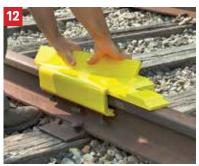
Test tightness of derail on rail.
