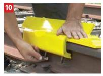
Hand-tighten thumbscrews on field side.
