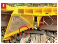
FOR WOOD TIES: Seat tie brace notch against the edge of the tie plate, a tie clip, or the edge of the tie.
