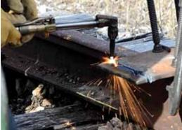
Mark each tie plate about an inch away from the rail base. Use a metal-cutting power saw or a torch. If using a saw, remove the spike on the gauge side and cut the plates. If using a torch, you will need to remove the two tie plates from under the rail, crop them, and then reinstall them under the rail, re-spiking the outer portions of the plates. Do not, as a short cut, permanently remove the tie plates. They are needed to support the rail and hold to gauge.
