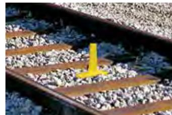
Attach Track Clearance Marker cone to steel base after pounding into ballast between ties.
