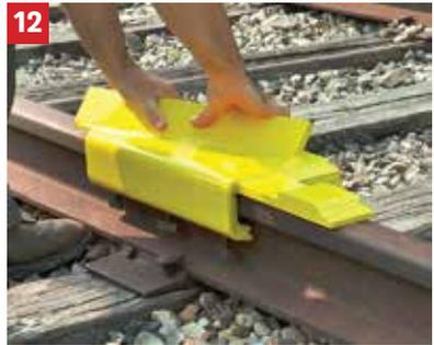
Test tightness of derail on rail.
