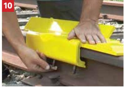
Hand-tighten thumbscrews on field side.
